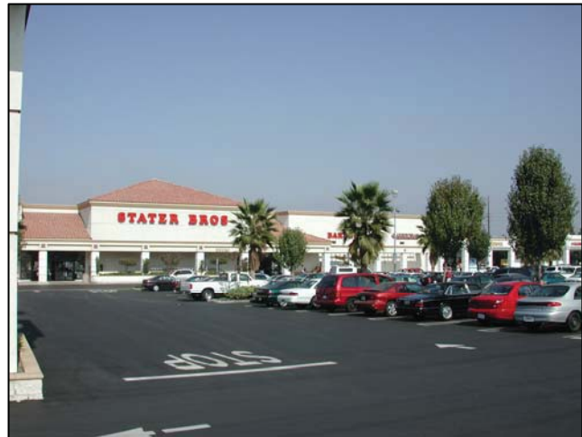
Retail center on Barton Road
